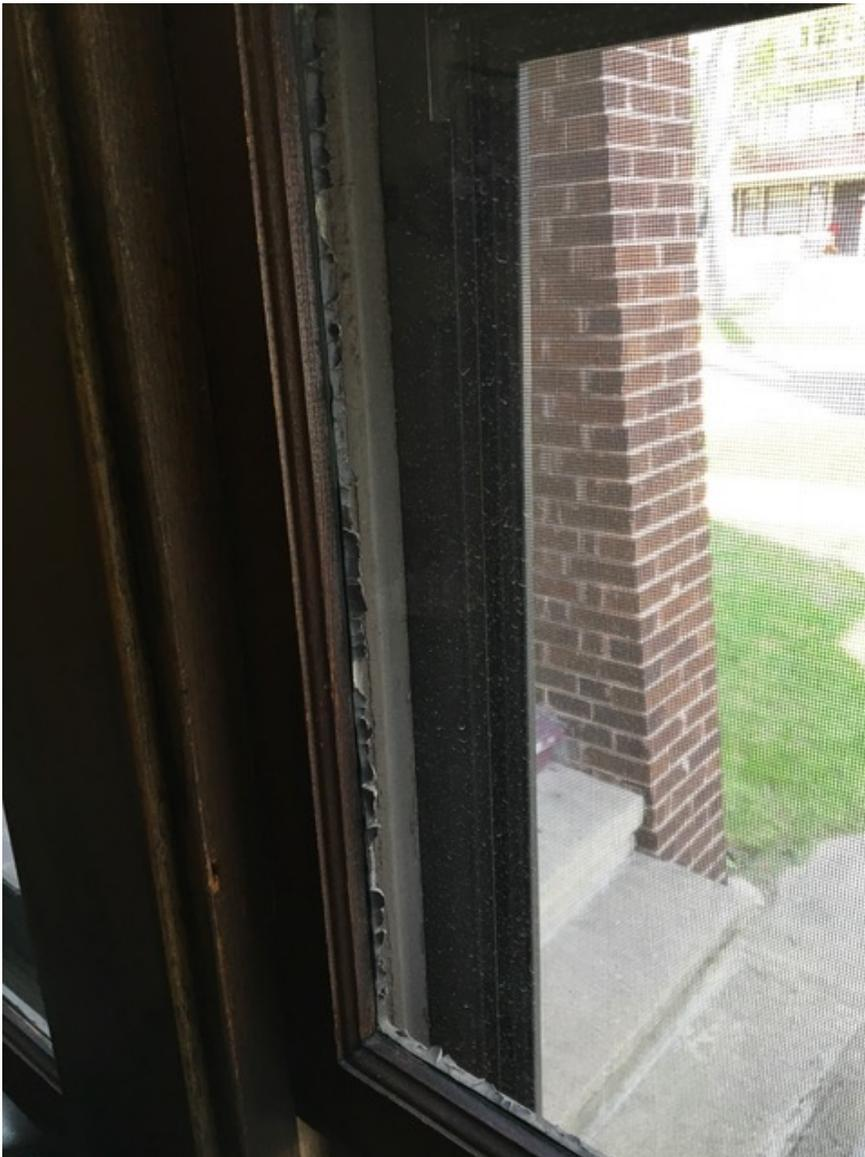
Space between windows and uneven sash where top window meets bottom results in major leak of cold air.
