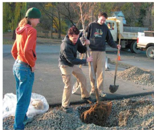
Relatively inexpensive, bare-root trees can be planted at grade and directly into CU Structural Soil parking lot base material by volunteers with no machinery. This method reduces project cost while obtaining superior performance of the system.
