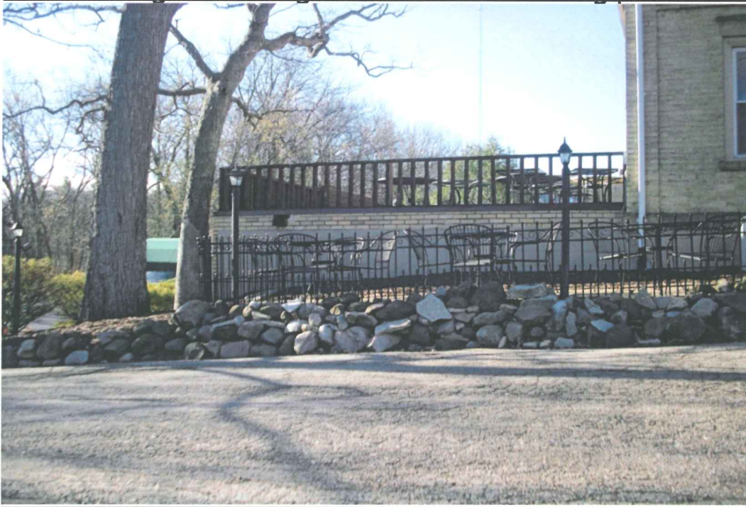
Outdoor on grade seating on south side of building (view from South) Outdoor Plaza deck above
