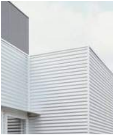
CORRUGATED METAL PANEL CONCEALED FASTENERS
