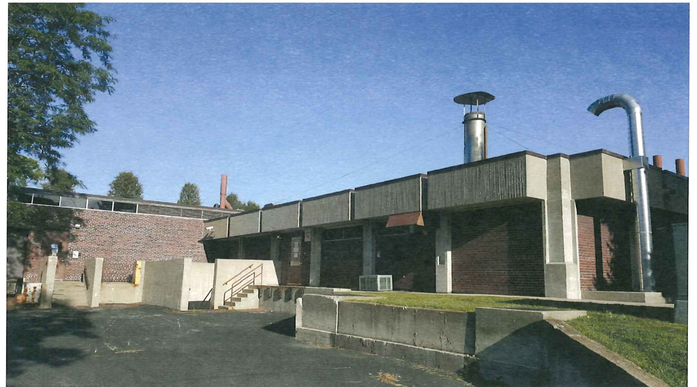
Southeast Loading facing Forward Drive
