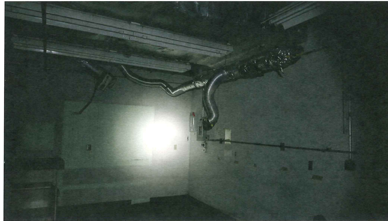
Lower Level Laboratory Space
