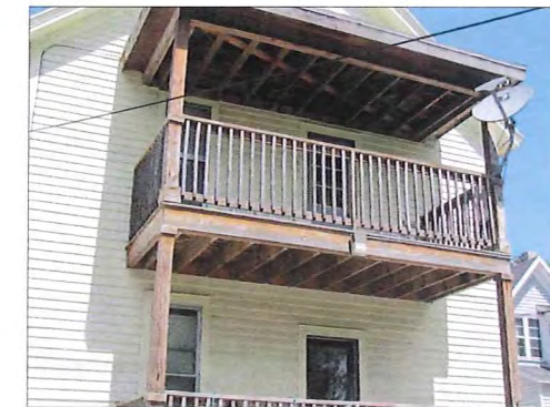
Exterior - Close Up - Back Porch
