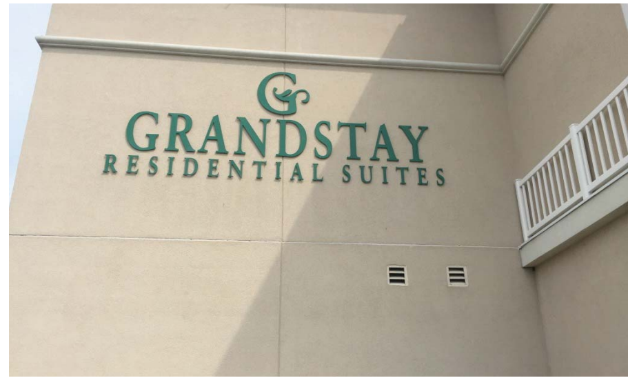
EXISTING SIGNAGE - WEST ELEVATION
