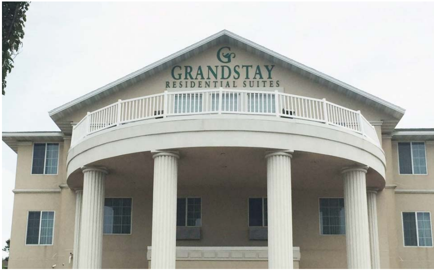
EXISTING SIGNAGE - NORTH ELEVATION
