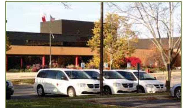
Existing structures (above)
