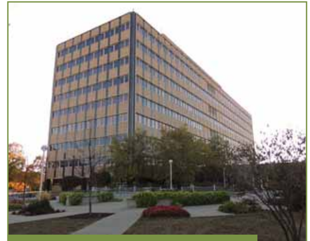
WiDOT northeast view
