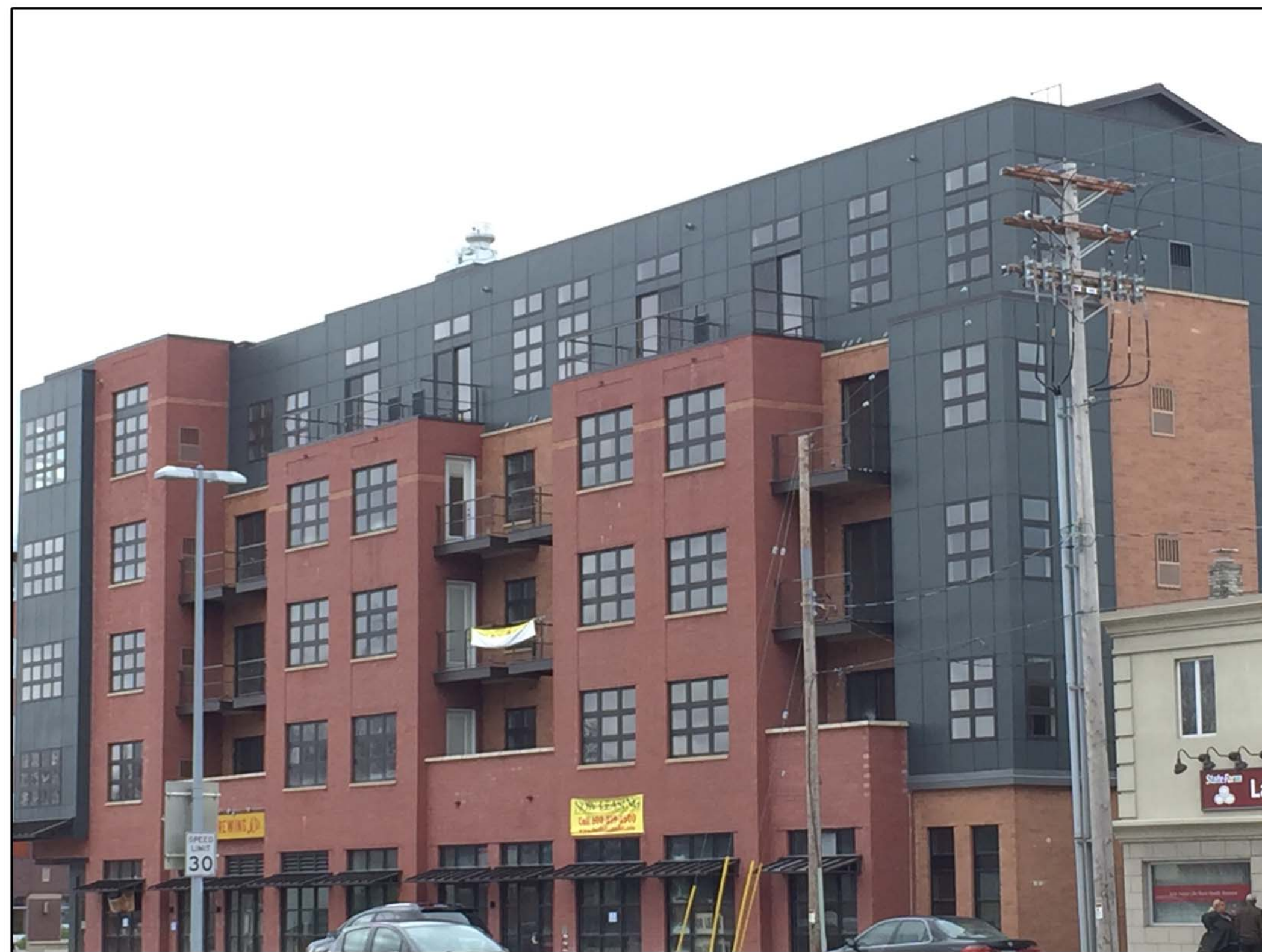
4. LOOKING FURTHER SOUTH ON PARK ST EXHAUST VISABLE
