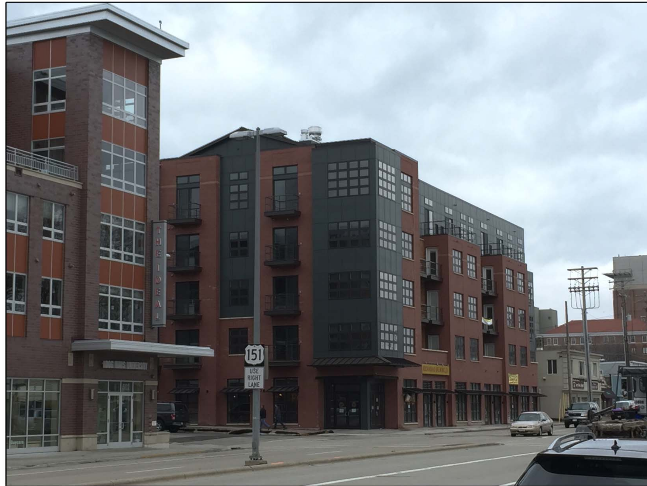
1. LOOKING NORTH ON PARK ST. EXHAUST VISABLE
