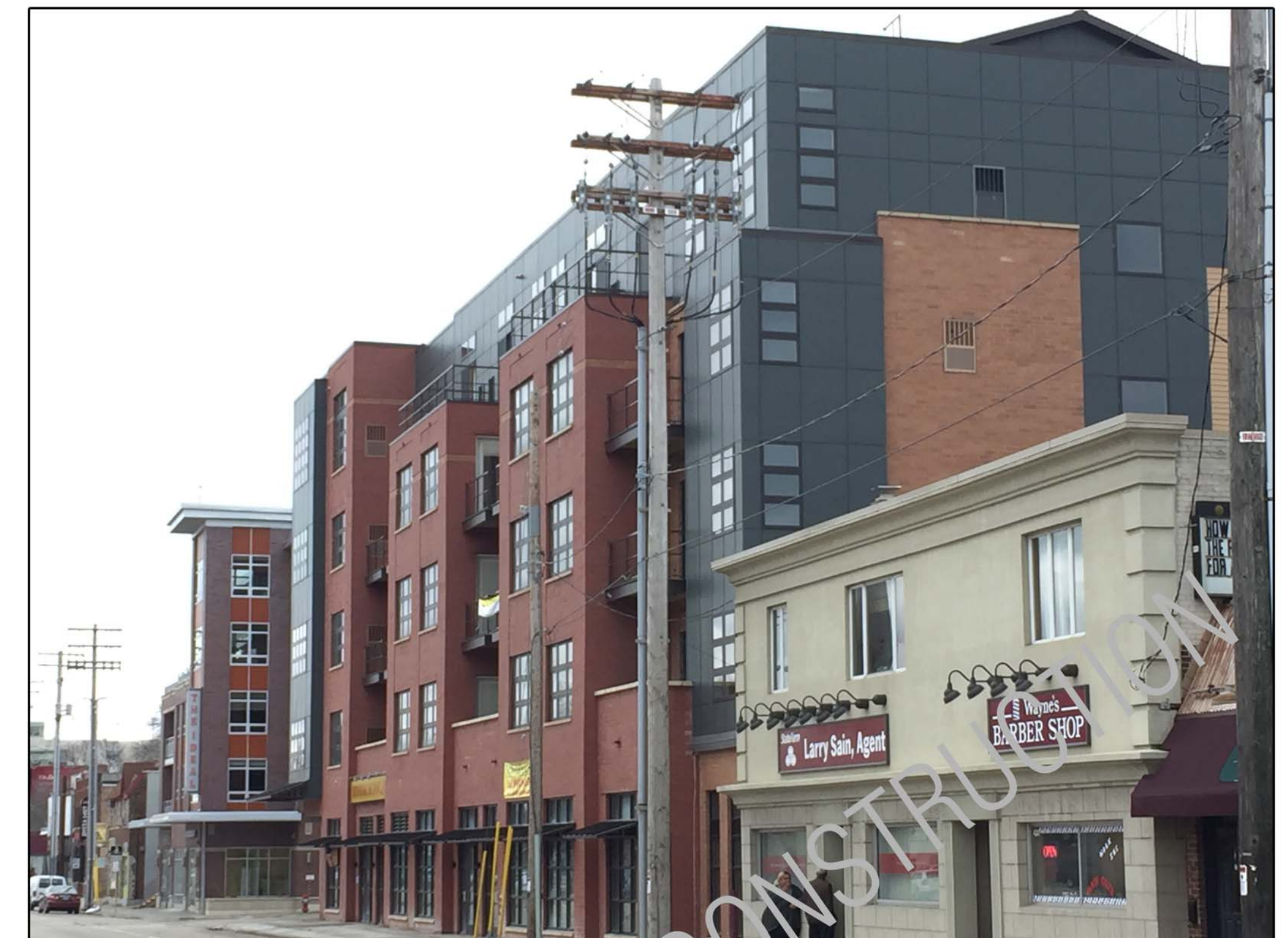
5. LOOKING SOUTH ON PARK ST EXHAUST NOT VISABLE
