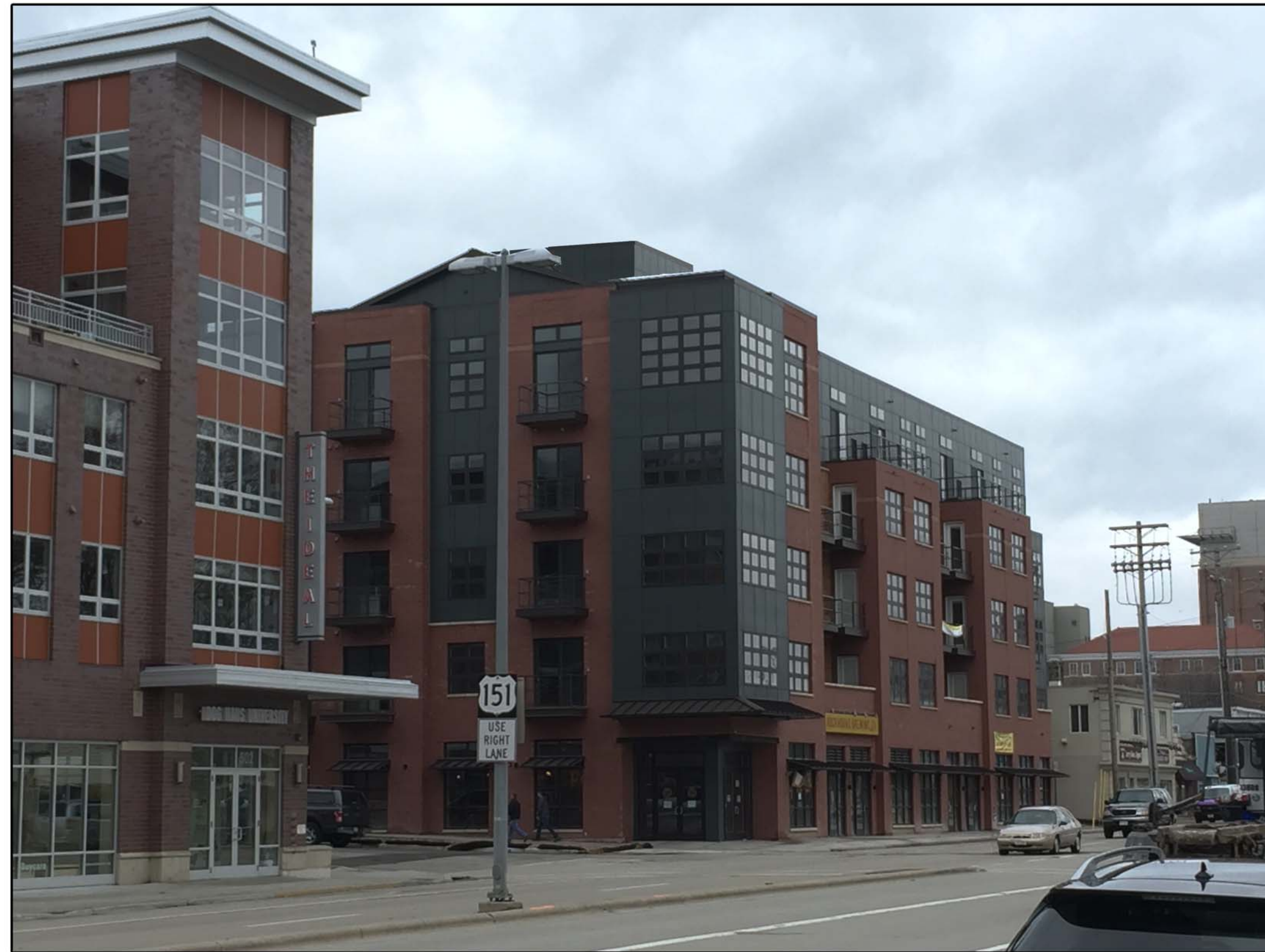
1. LOOKING NORTH ON PARK ST. EXHAUST VISABLE
