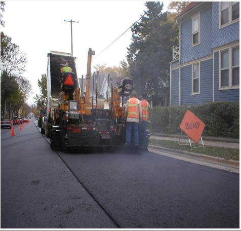
TACK COAT APPLIED TO LOWER ASPHALT LAYER
