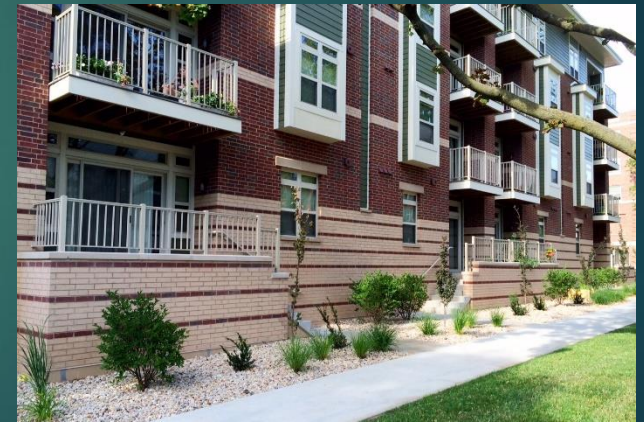
A building with a similar concept: The Vicinato at South Mills & Mound Street
