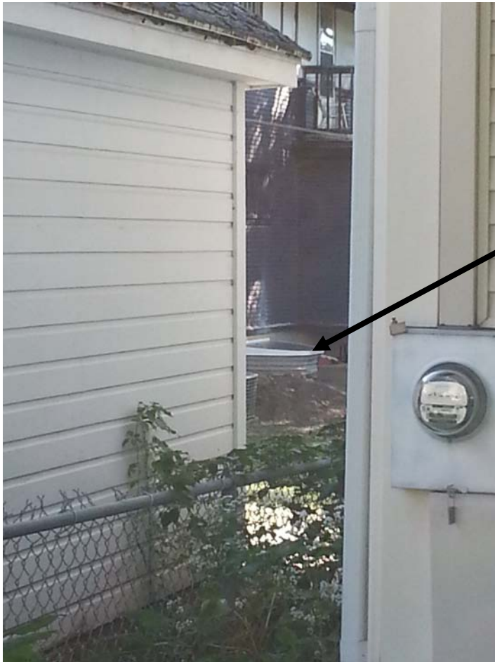
Photo by Building Inspector
