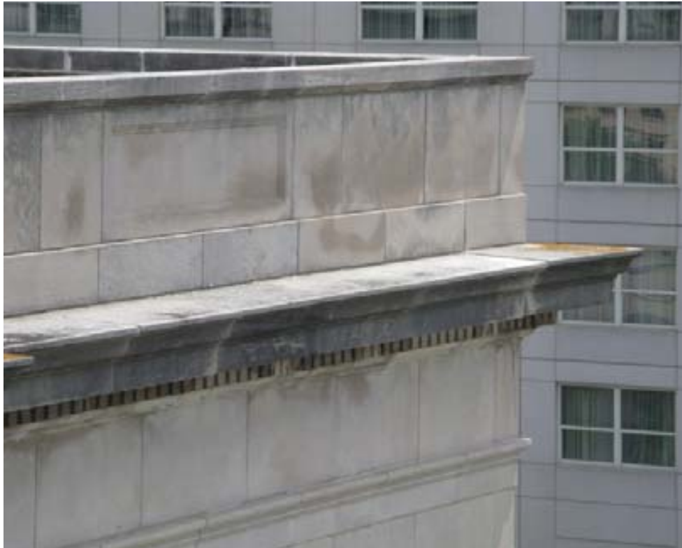
deteriorating mortar joints / mold
