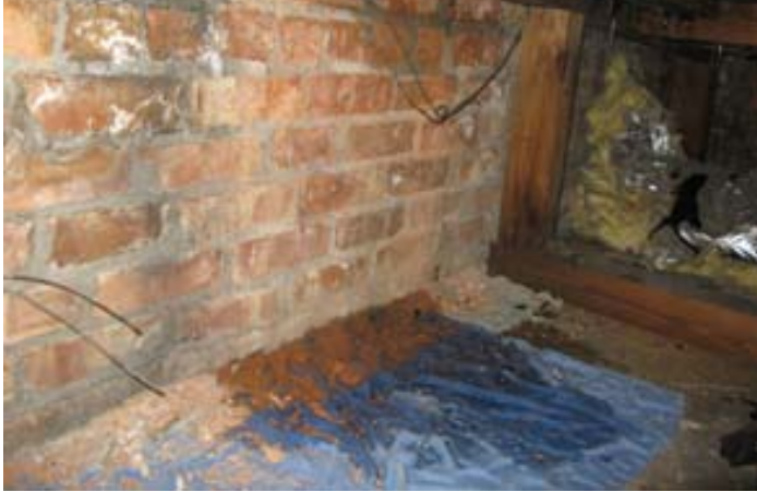
water infiltration
