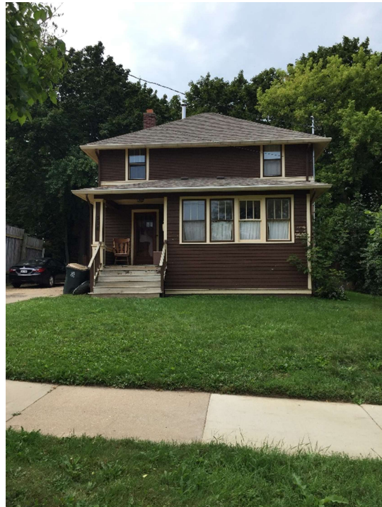
306 Lathrop, Front – East Elevation
