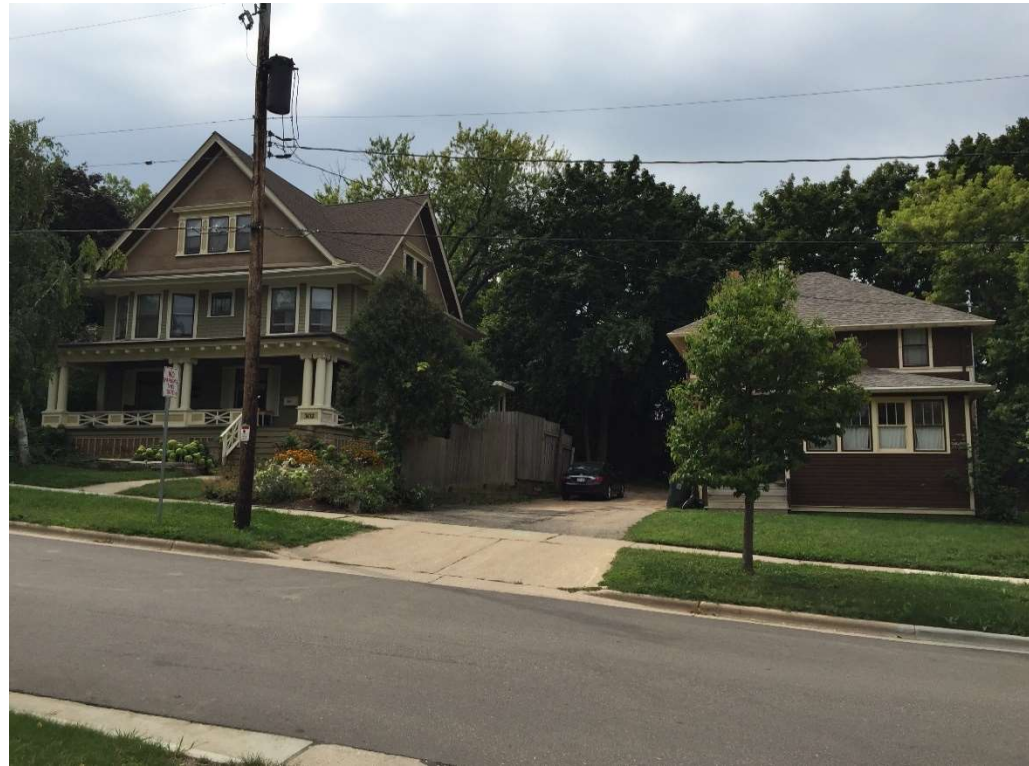
302 Lathrop on Left, 306 Lathrop
