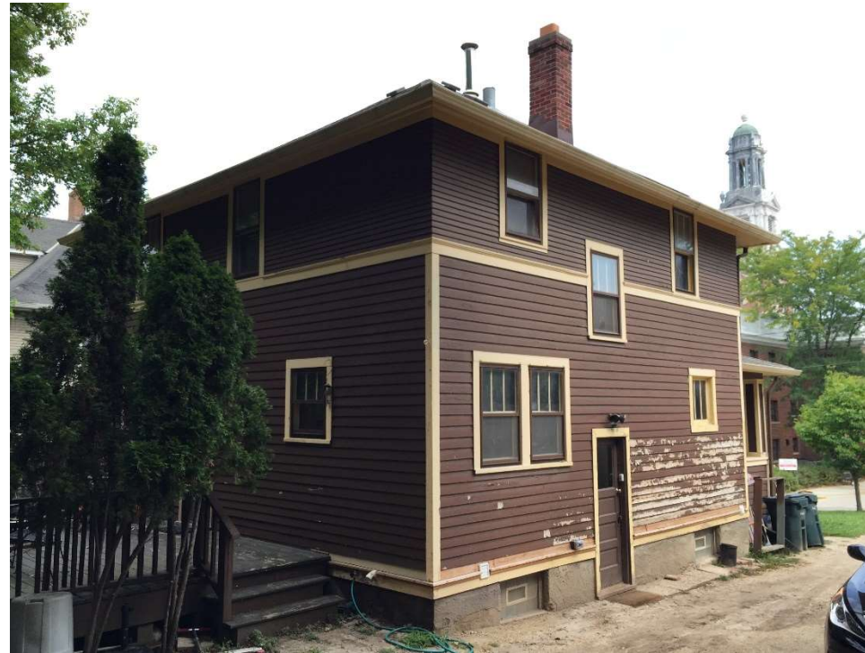
306 Lathrop, Side – Southwest Elevation
