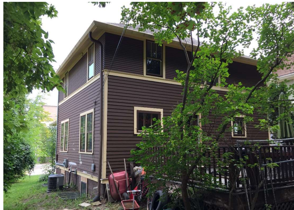
306 Lathrop, Northwest Elevation
