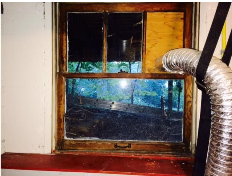
Inside of window #2. Note - The dryer vent (installed by previous owners) will be vented through the wall (not through the window).
