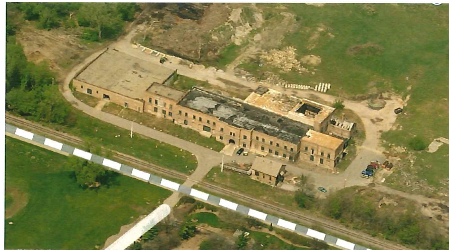
EXISTING SOUTH FACADE AERIAL
