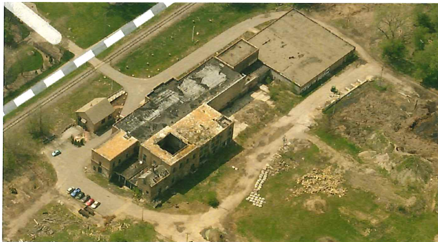
EXISTING NORTH FACADE AERIAL
