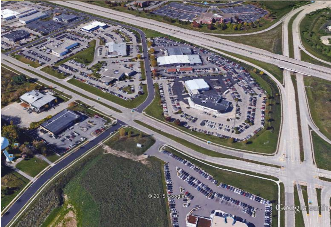
High Crossing Blvd.
