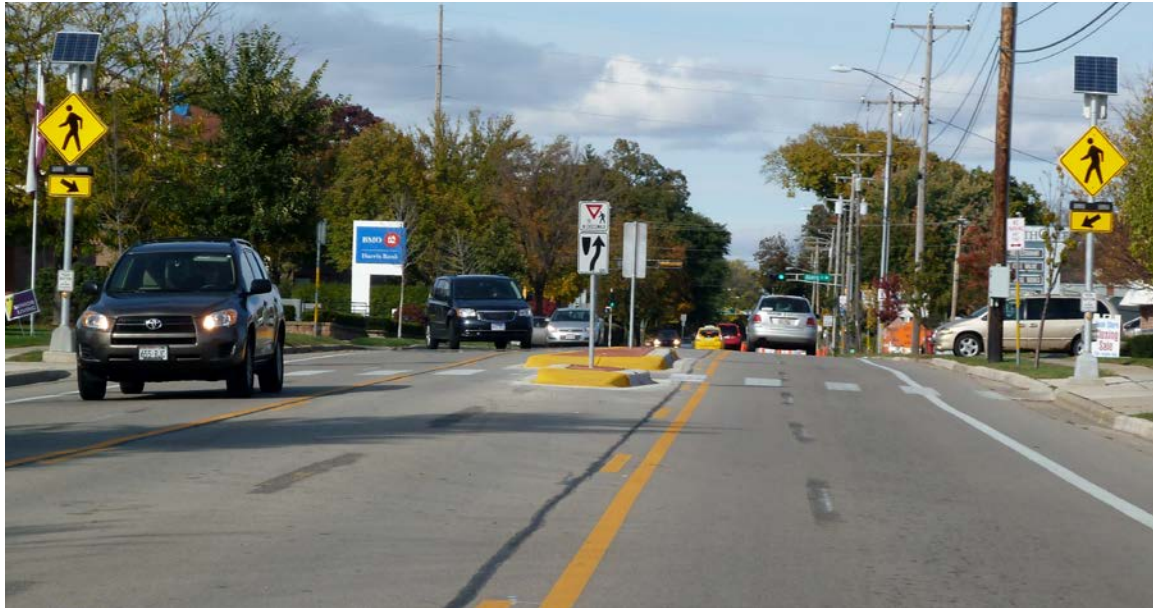
Image 2. Enhanced pedestrian crossing with RRFB at Northgate Shopping Center.
