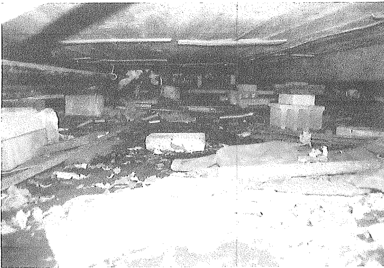
What passed for a foundation at 5980 Lake Edge, a collection of concrete blocks resting on wet soil. Note limited working room. Due to the soil and water table issues, a floating slab system was used to support the foundations. The framing was significantly twisted, but was not difficult to restore.
