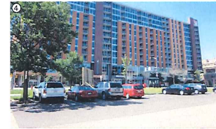
View from Proposed Site—Building Design to be Coordinated with City of Madison's Lake Street Reconstruction
