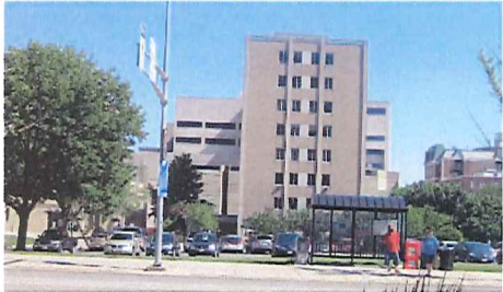
UW-Extension Building; Site of Possible Phase 3 Expansion
