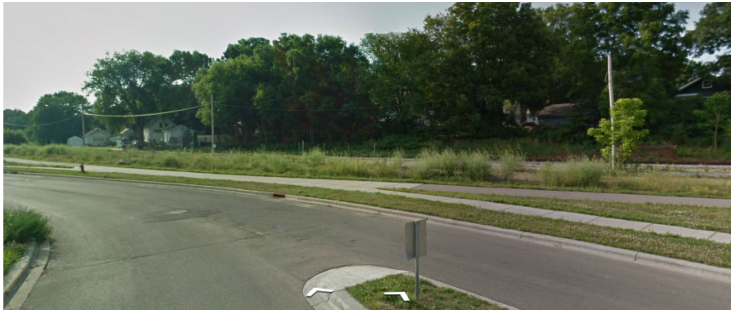
6th Street and Winnebago Street - Looking East
