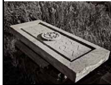
Existing Masonry and Stonework
