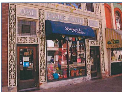
Castle and Doyle Building
