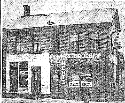
Here is pictured the building at the northeast corner of the intersection of W. Main and S. Bassett sts., which is the subject of today's article on Madison's historic buildings, by Alexius Baas.—Capital Times staff photo.
