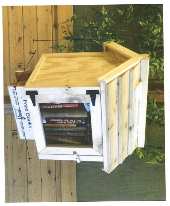
glass window. Materials: The Little Free Library is made of plywood and recycled barn wood, with a cedar roof and plexi-
