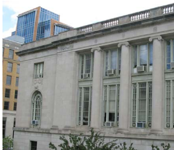
Figure 8 – 3 of 12 Partially Engaged Columns on the South Elevation
