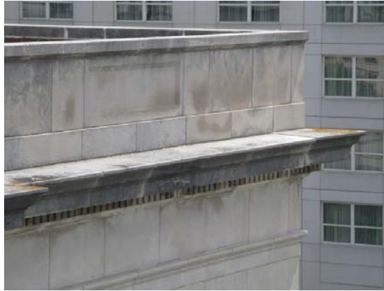
Figure 9 – Stone Cornice and Parapet
