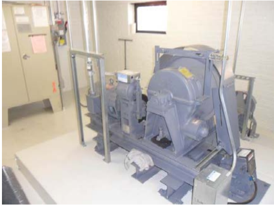
Figure 52 – Exposed Elevator Motor
