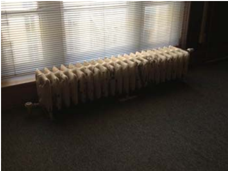
Figure 35 – Steam Radiator
