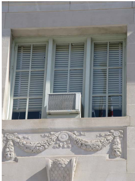
Figure 63 – Steel Window with Stone Carving Decorations
