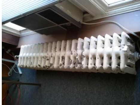
Figure 37 – Electric Window Air Conditioning Unit Installed
