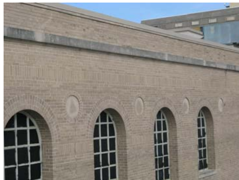
Figure 10 – Brick Façade in the “U” Shape
