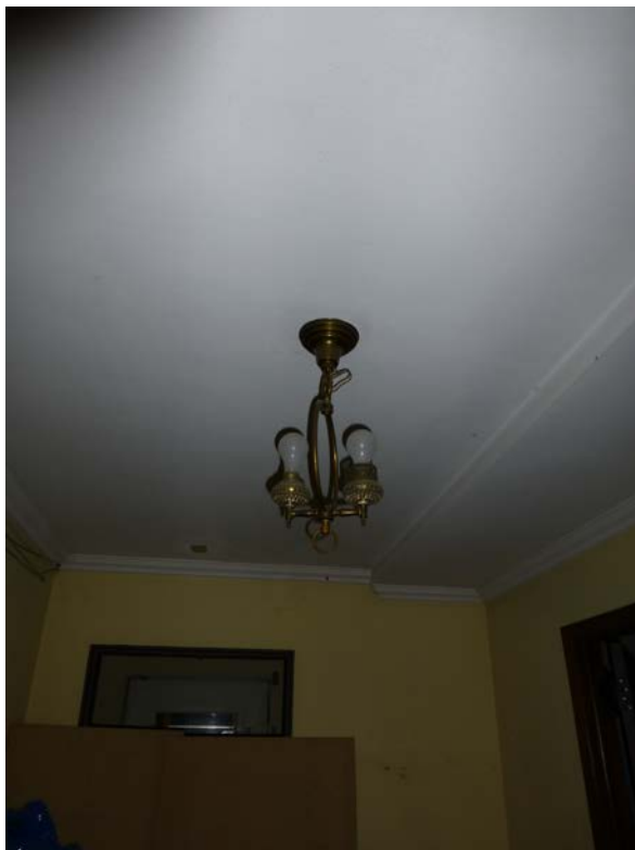
Image 10 Original light fixture, main entry, first floor
