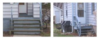
front porch is missing door; garage is leaning and has chipped paint.
