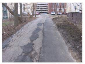
Asphalt problems in Sections B Alley (poor condition)
