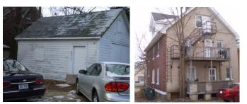
garage has chipping paint, roof damaged, mold
