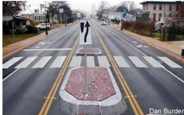
Figure 9. Pedestrian Safety Island
