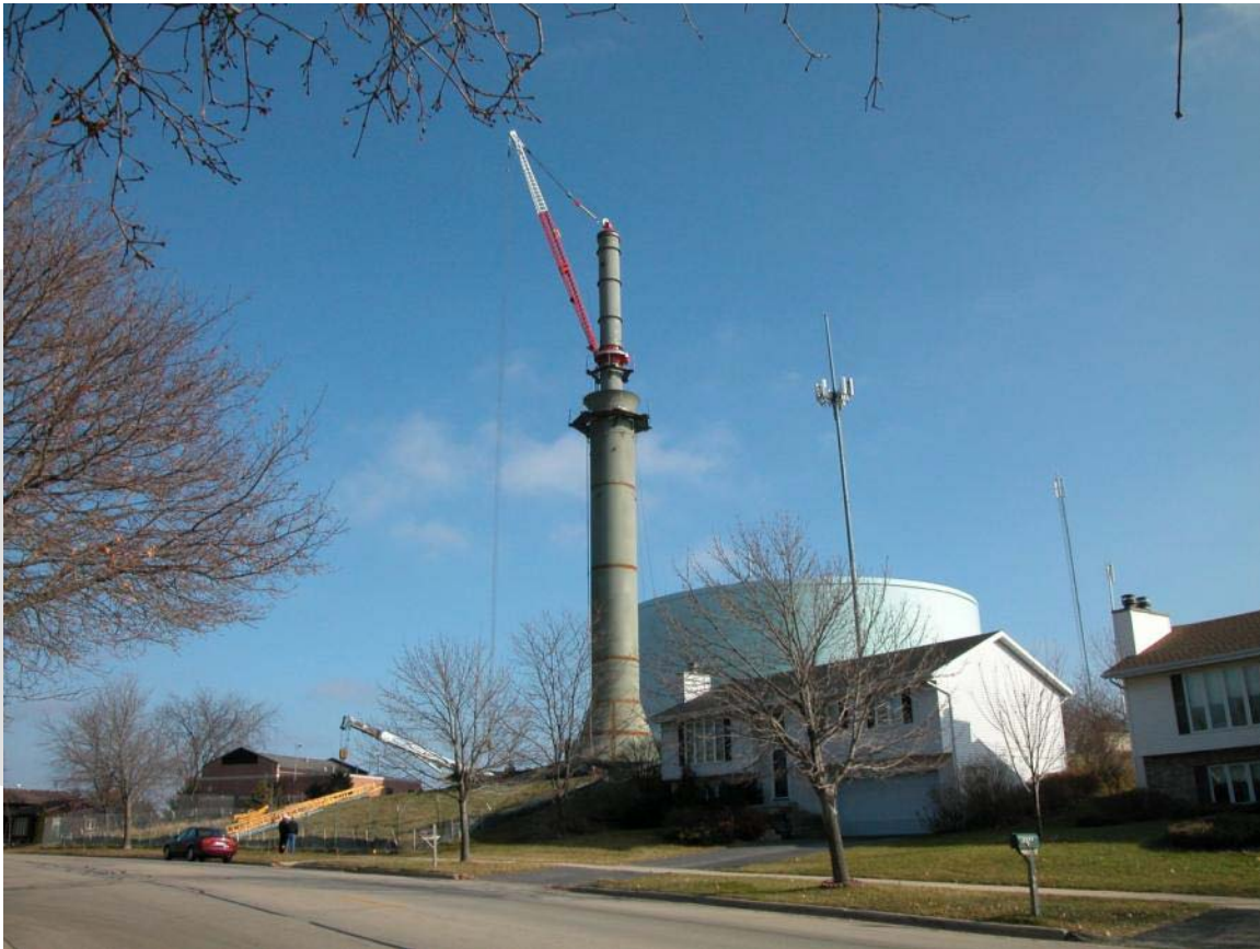
TOWER UNDER CONSTRUCTION, NOVEMBER 2011
