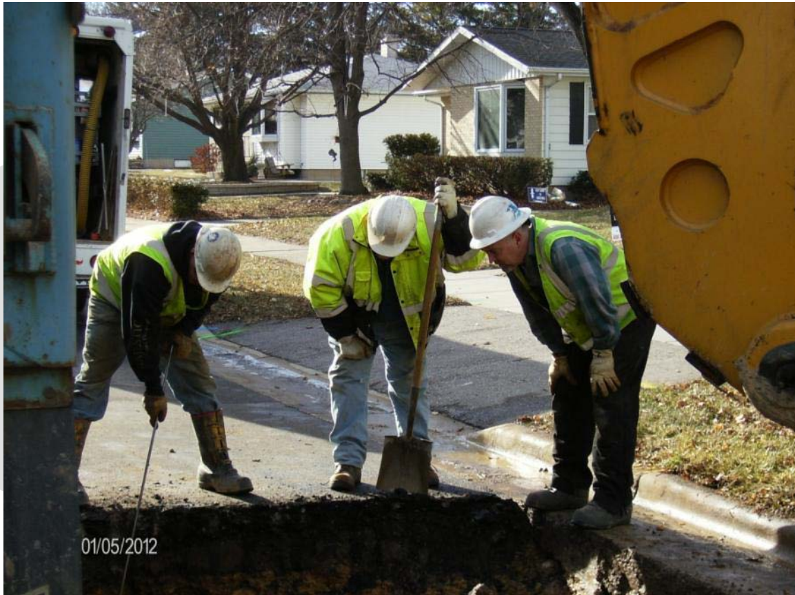
MWU CREW MEMBERS REPAIRING A WATER MAIN BREAK
