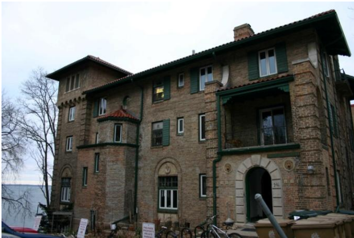
146 Iota Court – scale and character of most buildings in area
