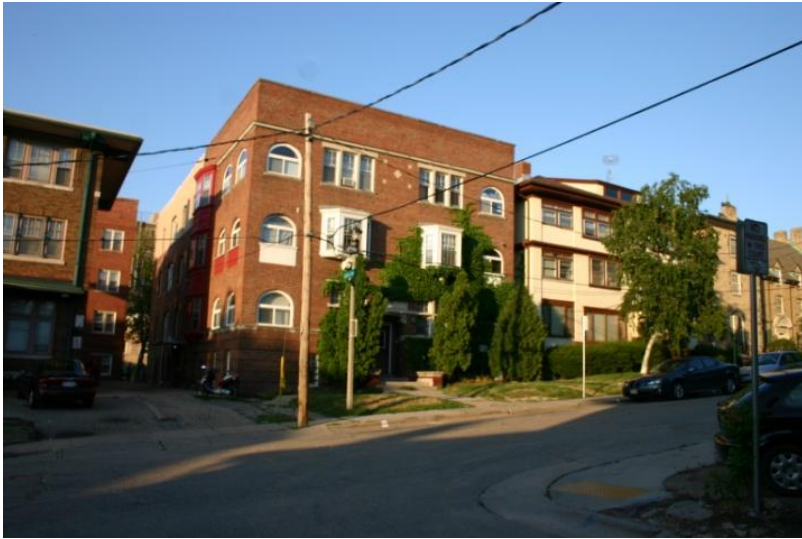
619 N. Henry – proposed for demolition
