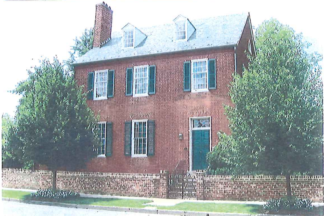
Restored exterior shutters, windows and trim with original finishes
