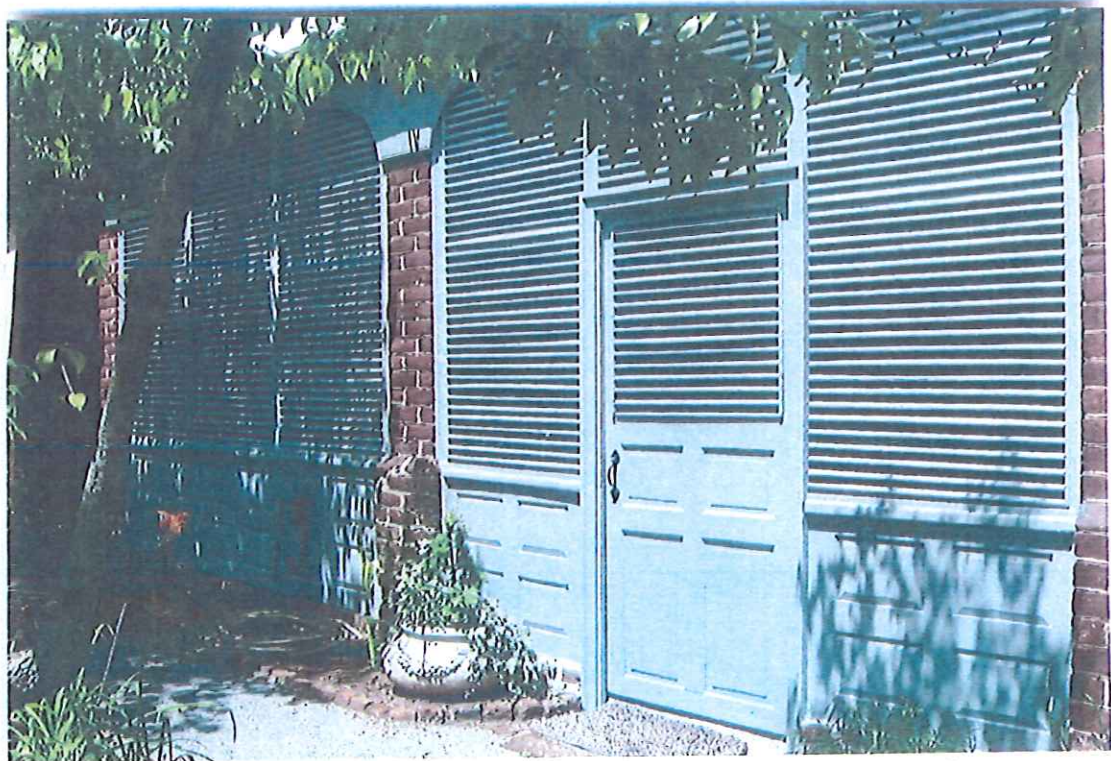
Restored louvered lean-to (west side), one of two extant originals in the City of Fredericksburg
