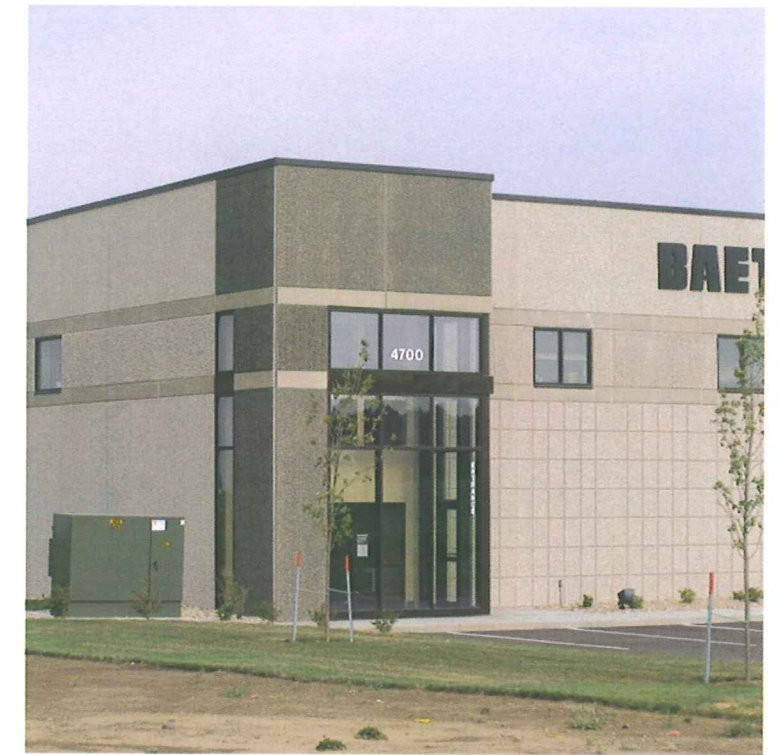
Examples of precast panel finishes. The face finish will provide tone and color variation.
