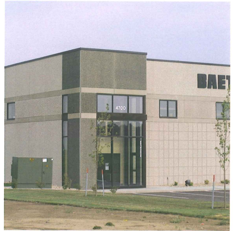
Examples of precast panel finishes. The face finish will provide tone and color variation.
