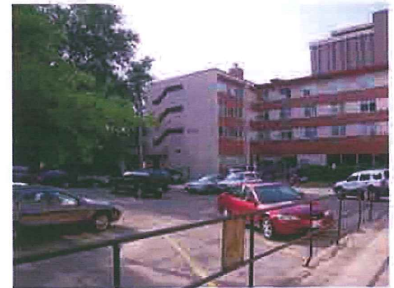
1001 University Development. Existing Conditions
