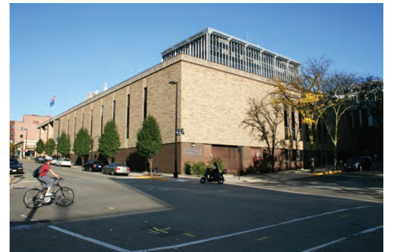
VIEW FROM MIFFLIN STREET AND HENRY STREET
