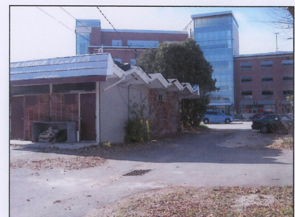
NORTHEAST CORNER OF LOT LOOKING SOUTHWEST
