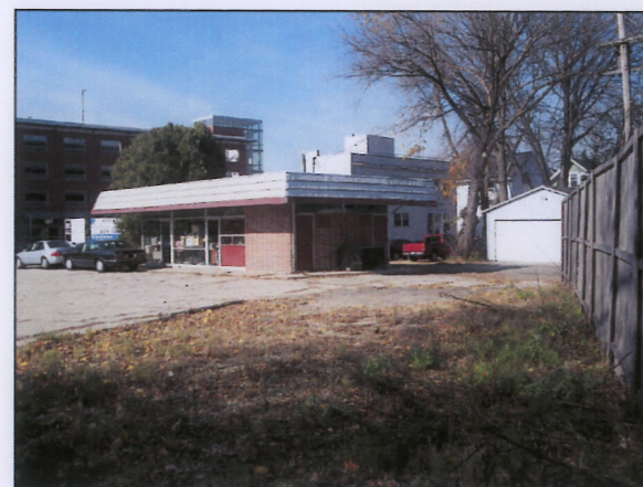
WEST CORNER OF LOT LOOKING NORTHWEST
