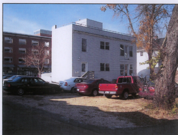
CENTER OF ALLEY LOOKING NORTHWEST
