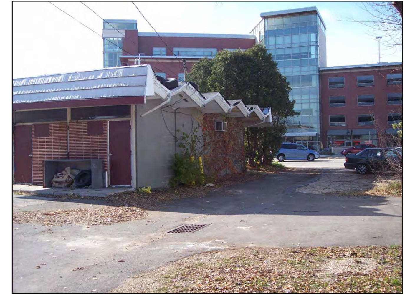
NORTHEAST CORNER OF LOT LOOKING SOUTHWEST
