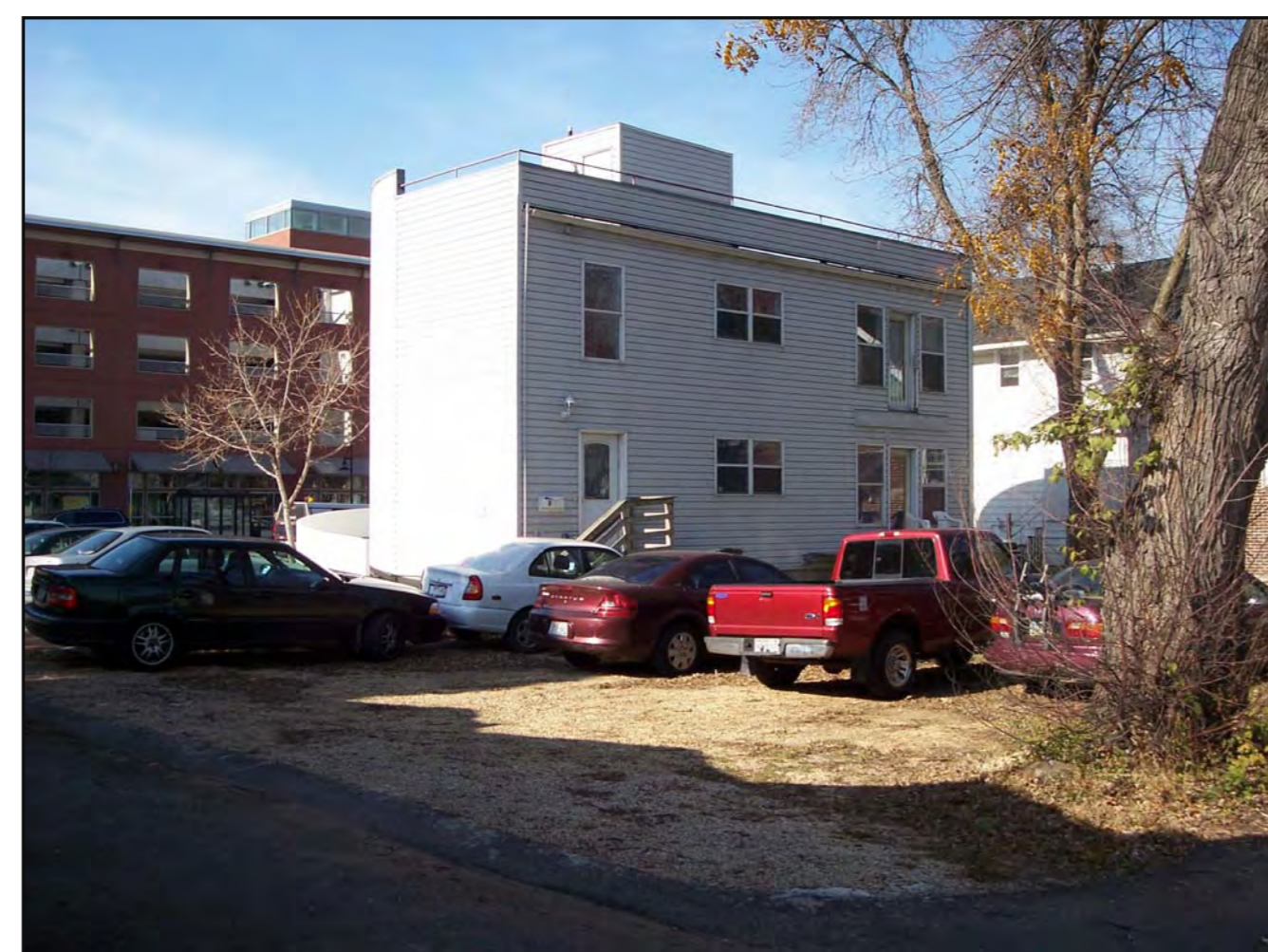
CENTER OF ALLEY LOOKING NORTHWEST
