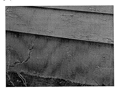
• As a result of their age, the homes are showing signs weathering and need to be completely pressure washed and repainted.
