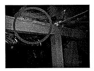
• Two of the three poured-wall foundations are showing signs of possible water infiltration. Lack of exterior basement waterproofing is the probable cause.
