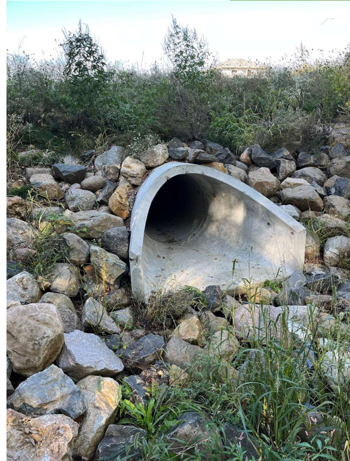
Outfall in dry weather
