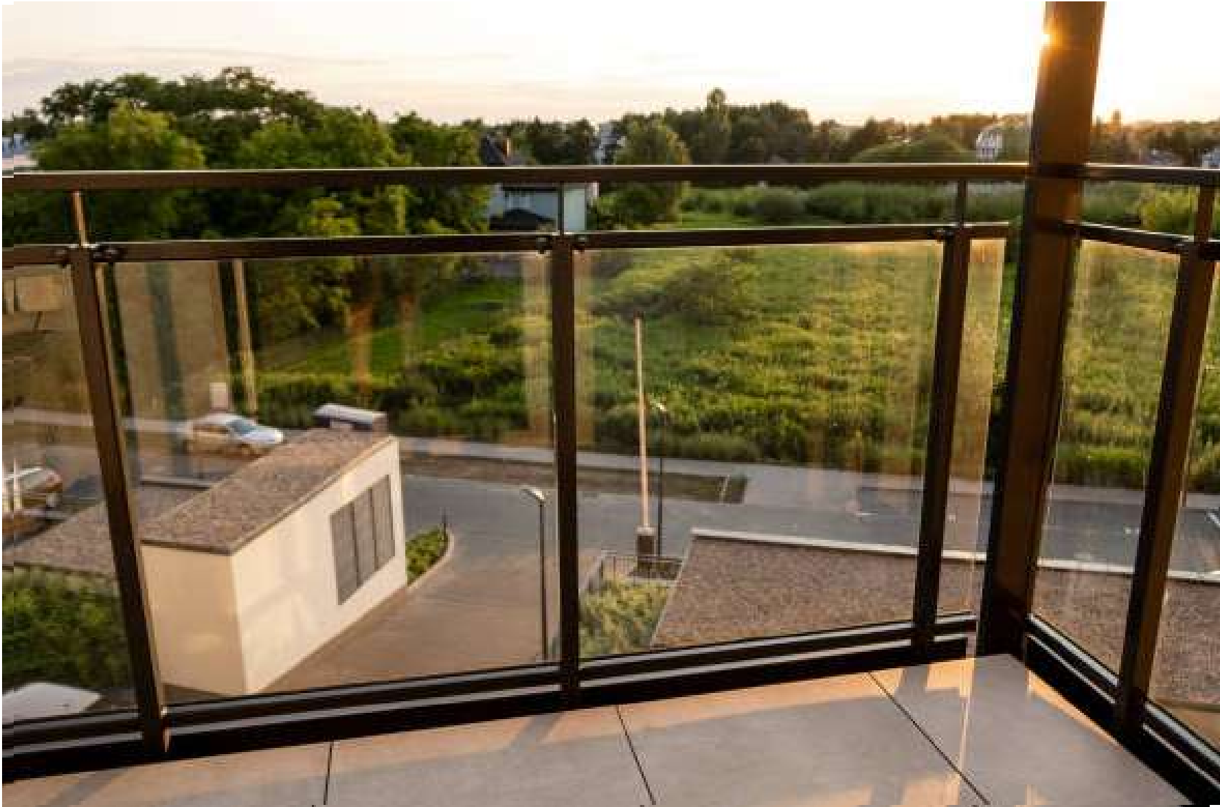
GLASS RAILINGS (EAST ELEVATION)
