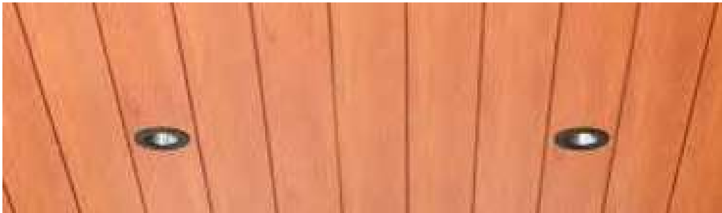
METAL SOFFIT (FIRST FLOOR CANOPY)
