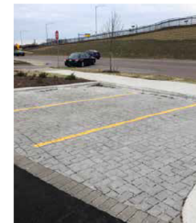
Pervious pavement at Portillos at West Towne.
