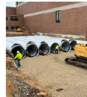
An underground stormwater detention system at West High in Madison.
