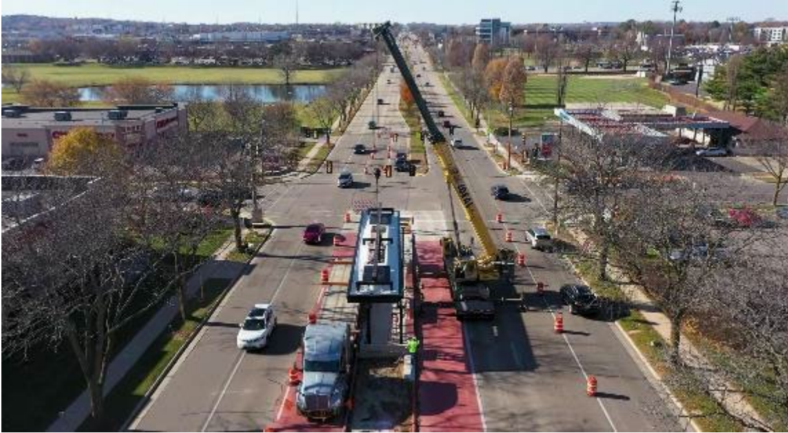
Figure 25 Erection of a Mineral Pt Rd BRT shelter. Photo courtesy of Wisconsin State Journal
