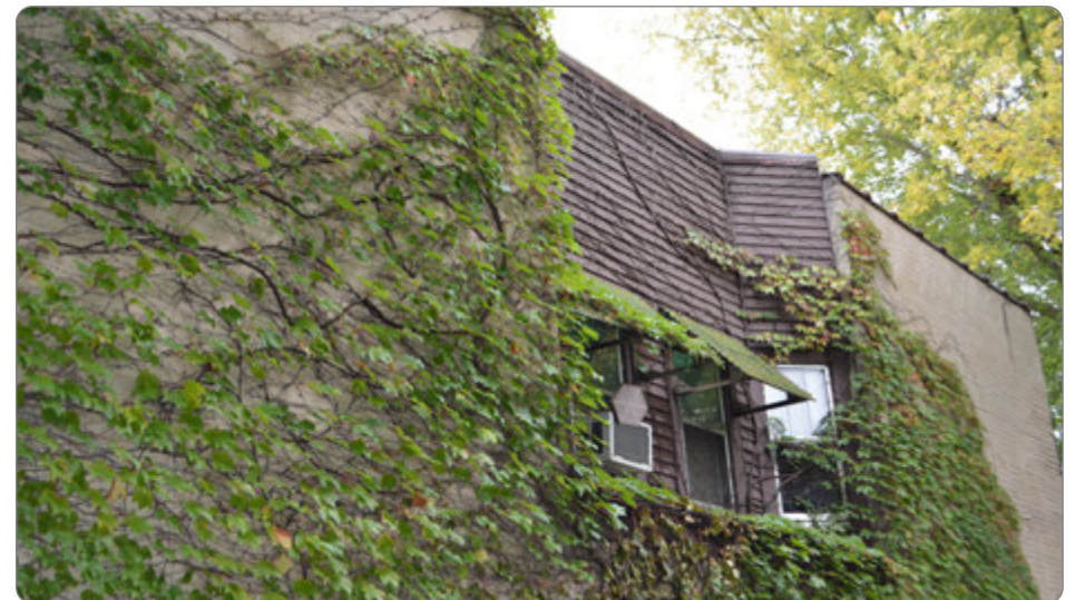
Figure 21: Growing vegetation that should be removed (41.23.3.d.2).
