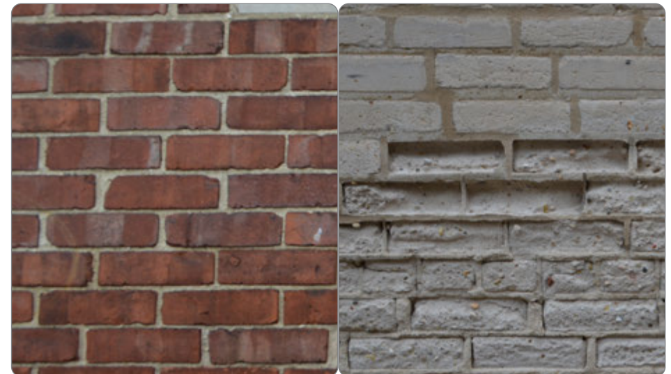
Figure 38: Proper vs. improper mortar alterations (41.24.2.a.1).
