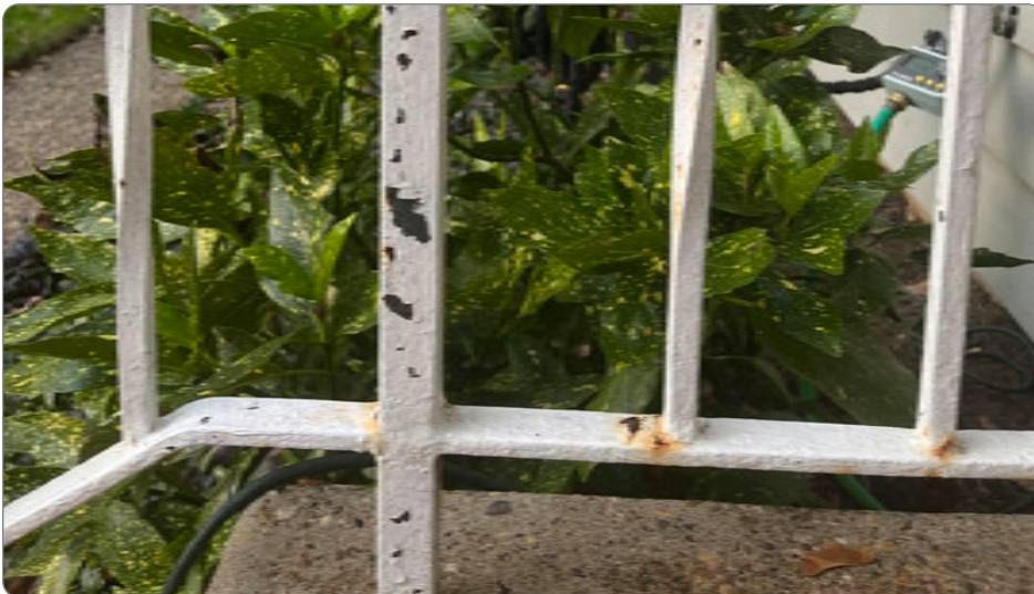
Figure 19: Examples of metal detailing which should be non-abrasively cleaned and repaired (41.23.3.c.1).
