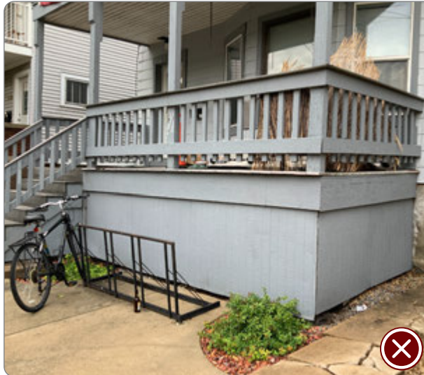
Figure 76: Example of a porch with no openwork design for ventilation (41.25.6.b.3).
