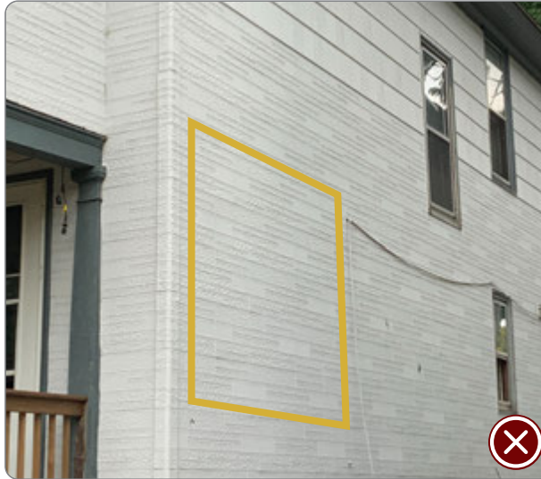
Figure 45: Incompatible replacement of historic siding (41.25.1.b.1).
