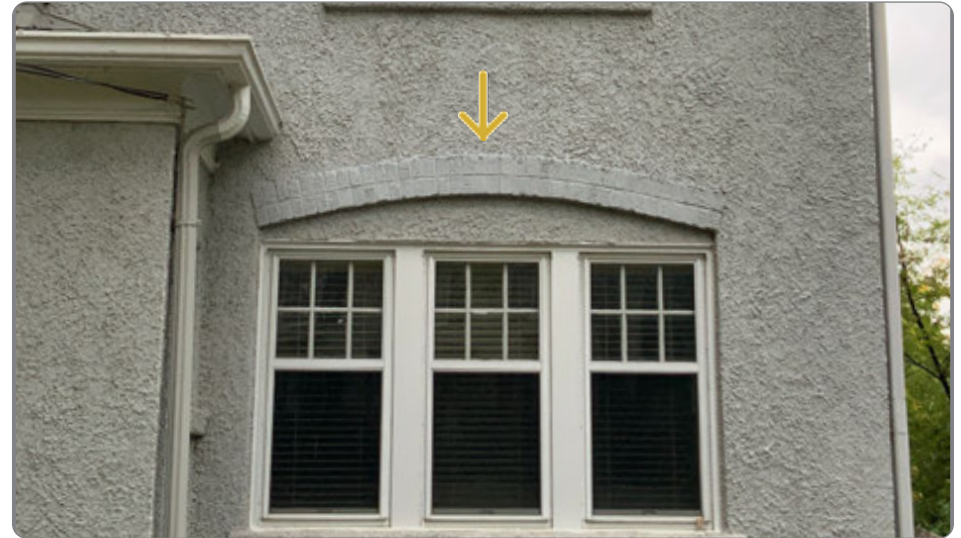
Figure 63: Infilled head above windows (41.25.5.b.1).
