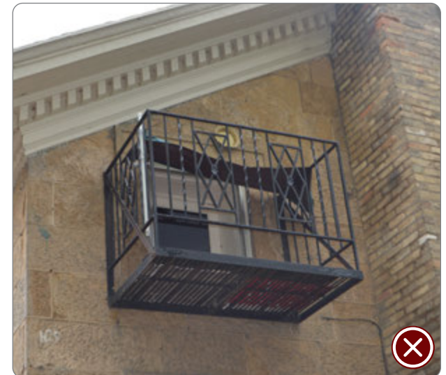
Figure 115: Incompatible balcony addition on front elevation (41.26.6.b).
