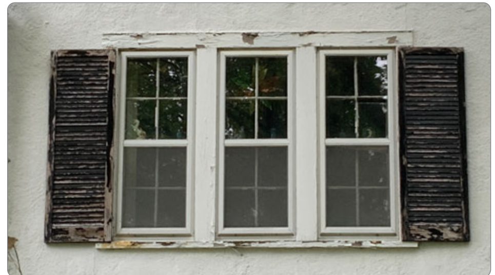
Figure 18: Example of wood shutters and window framing needing to be appropriately re-painted (41.23.3.b.1).
