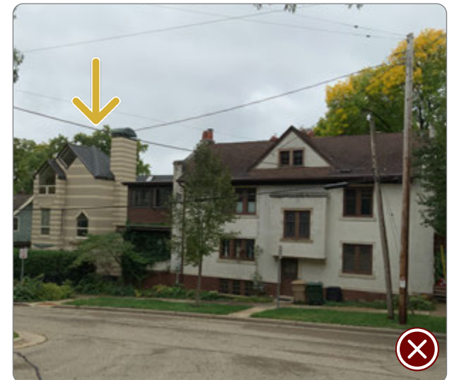
Figure 131: Infill construction demonstrating incompatible wall material (41.27.3.a.1).
