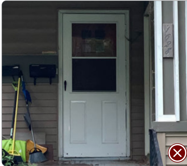
Figure 70: Example of an incompatible storm door. New storm doors need to be full light (41.25.5.d.3).
