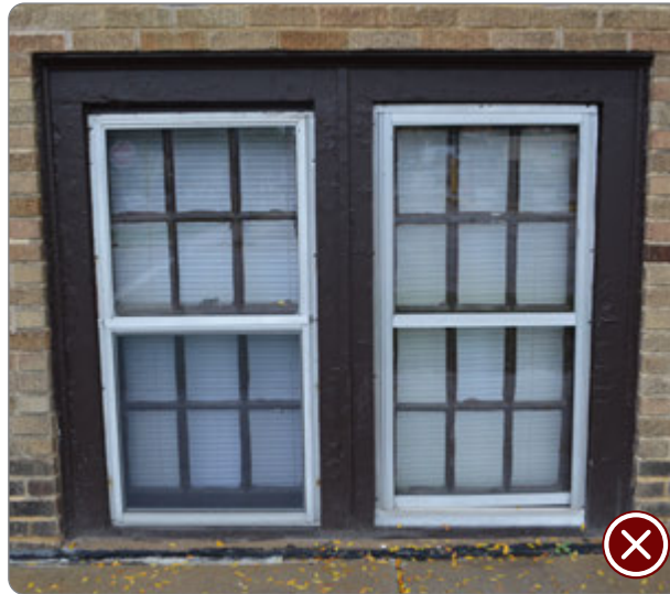
Figure 67: The left image has compatible wood framed storm windows with painted trim to match original sashes. The right image has incompatible reflective aluminum framed storm windows that do not blend with the historic sashes (41.25.5.c.6).
