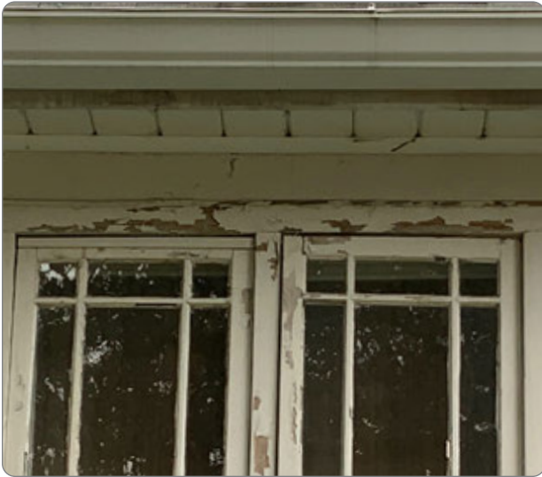
Figure 39: Wood features requiring repair (41.24.2.b.1).
