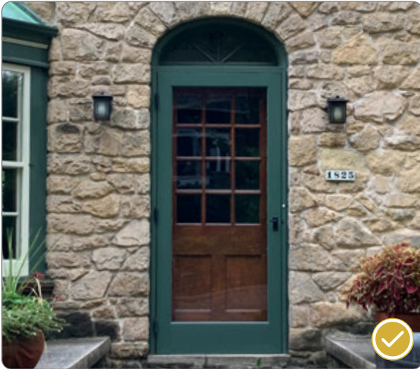
Figure 105: Compatible storm door (41.26.5.d.1).
