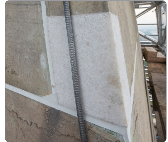
Figure 34: Example of a dutchman repair.
