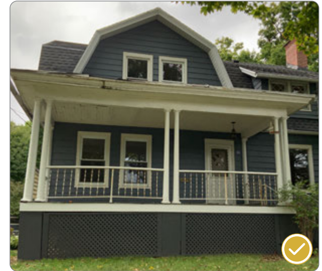
Figure 110: Example of a porch with compatible lattice for ventilation (41.26.6.a.2).
