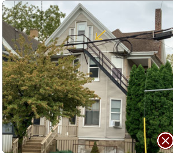
Figure 109: Example of a second exit stairway off the front of the building (41.26.6.a.4).
