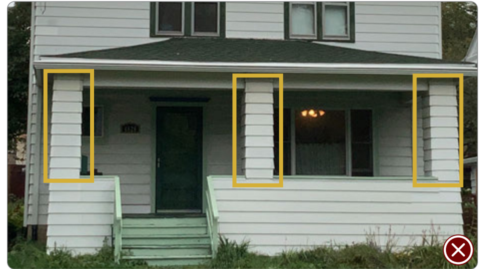
Figure 54: Incompatible wrapped wood columns (41.25.3.b.4).
