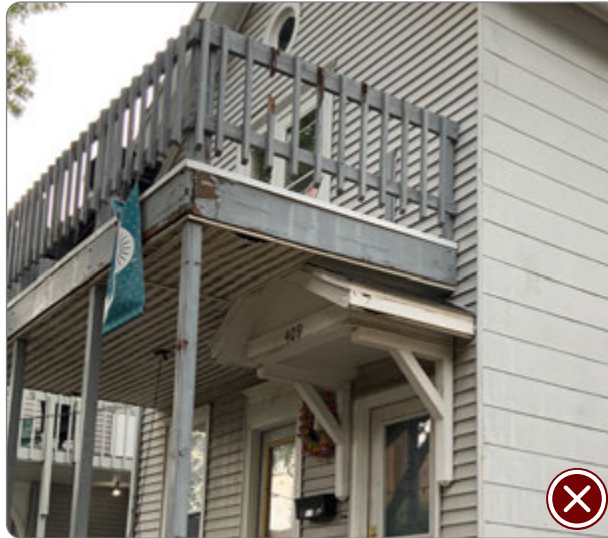
Figure 113: Incompatible balcony addition with out of character railing balusters and the deck cutting off the top of the gabled portico over the door (41.26.6.b).
