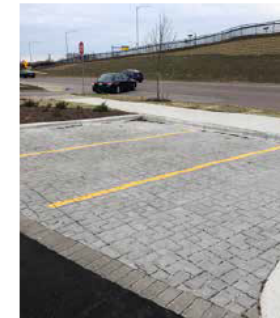
Pervious pavement at Portillos at West Towne.
