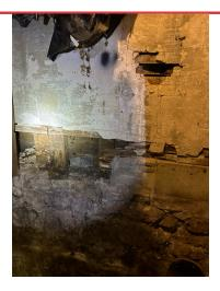
**ISSUE 7** Crumbing stone foundations. Rotten structural walls.
