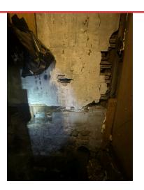
**ISSUE 5** Crumbing stone foundations. Rotten structural walls.
