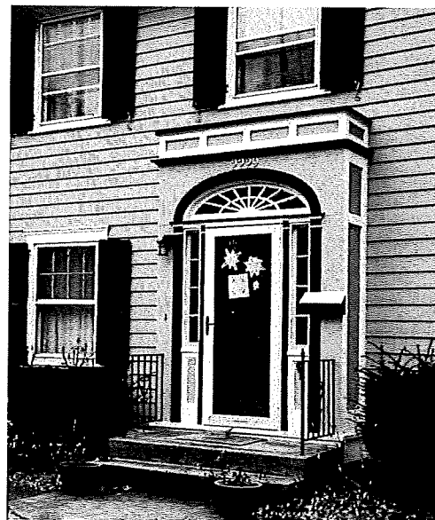
Front entrance looking southeast
