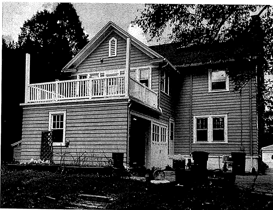
Rear view looking northwest. 2229 Eaton Ridge, 2023.
