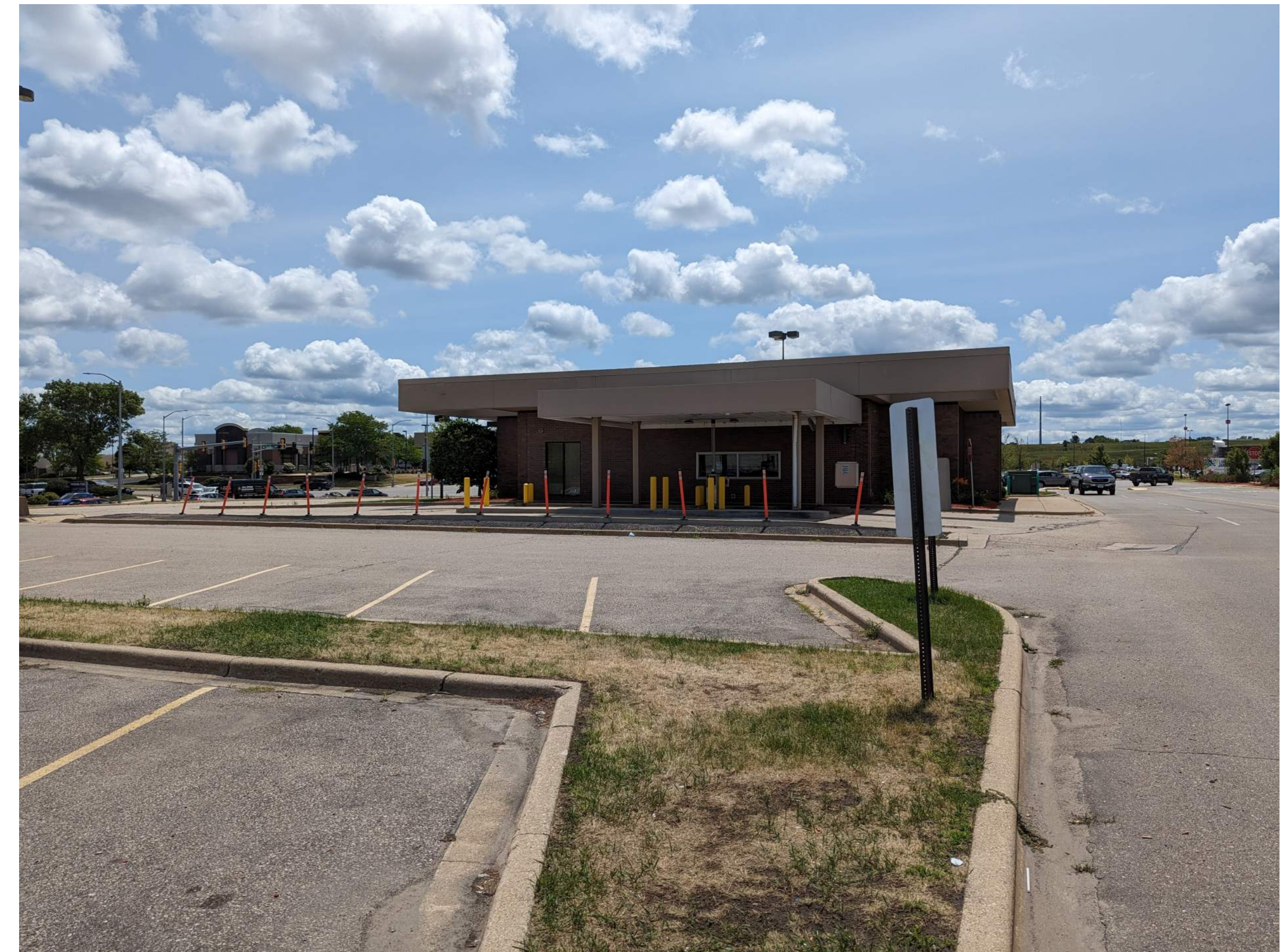
EXISTING NORTH ELEVATION OF CURRENT PROPERTY
