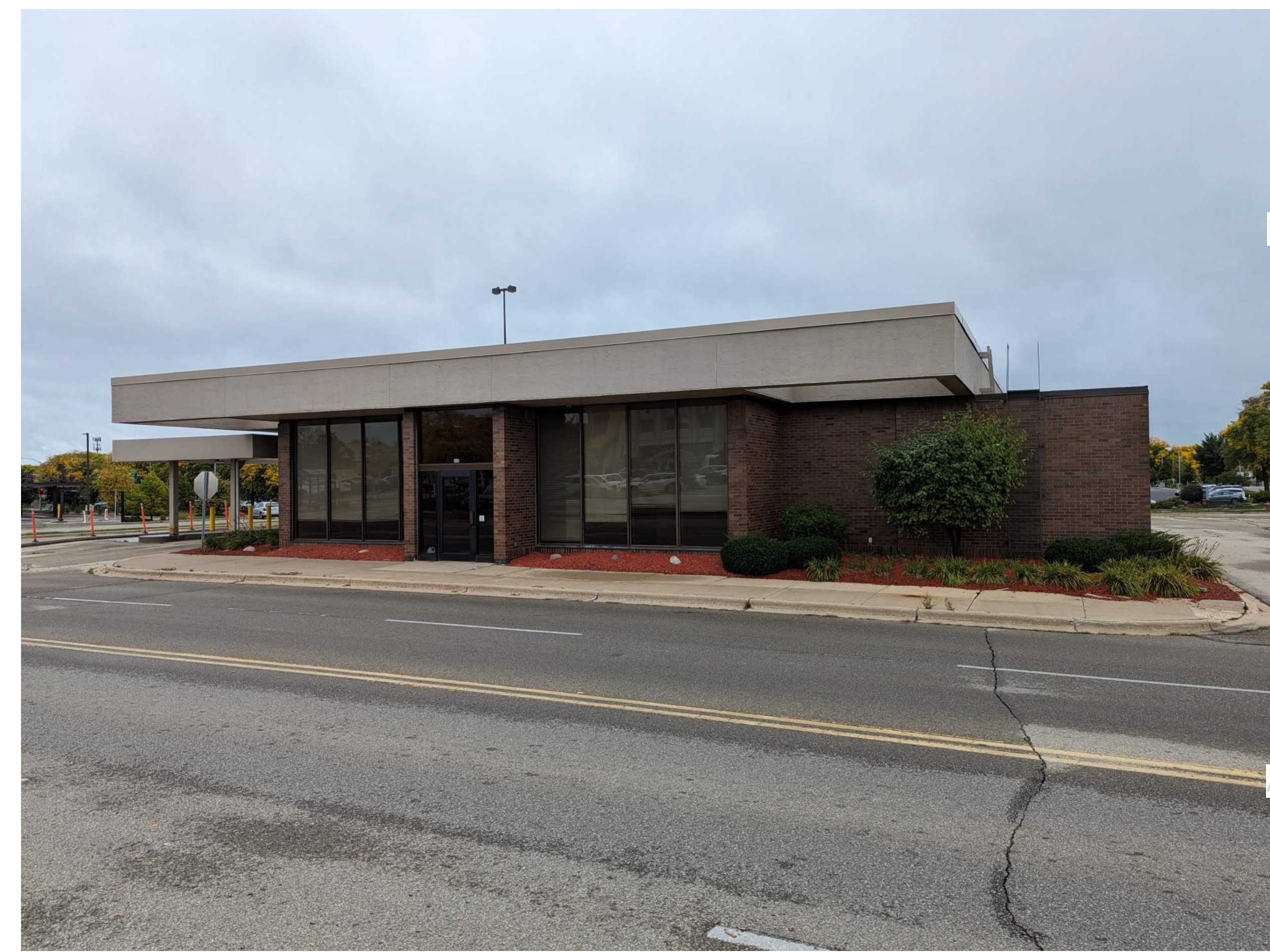
EXISTING WEST ELEVATION OF CURRENT PROPERTY
