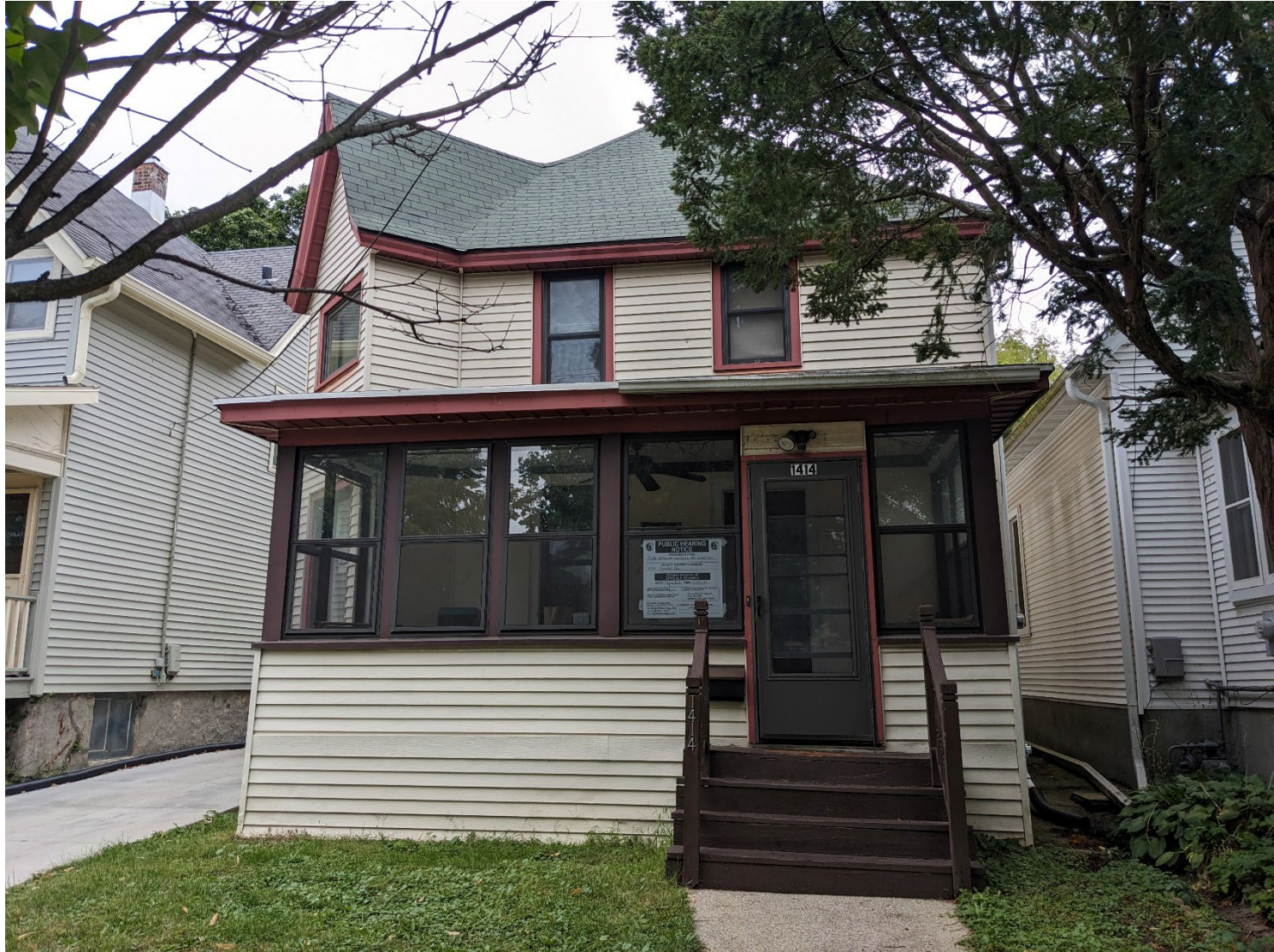
South Front Elevation – View from Jenifer St
